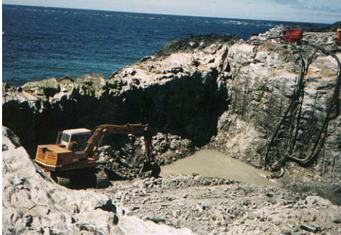
Figure 9. Site Part Excavated
