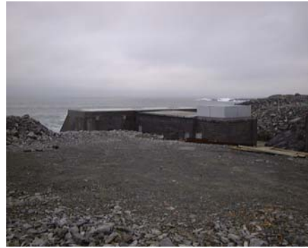
Figure 18. External View of Complete Plant
