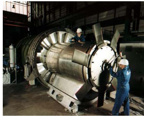
Figure 14 Turbine & Generator during Assembly
