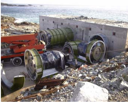
Figure 16. TG System Part Assembled at Site
