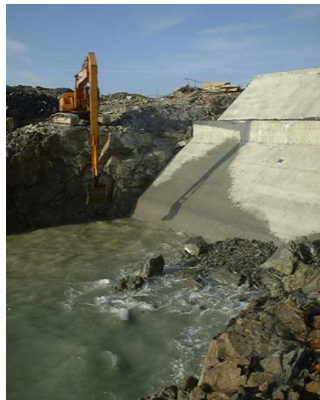
Figure 11 Excavating Debris from Wave Wall
